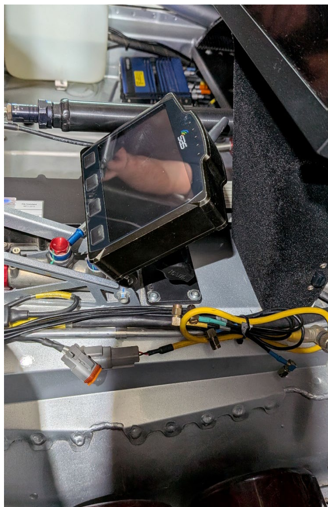
Figure 2. Unit mounted to the tunnel
